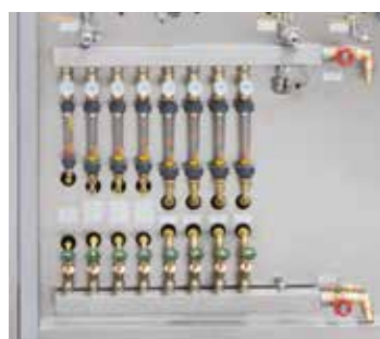
Cooling water distribution
