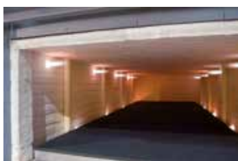
Furnace chamber with eight high-speed burners
