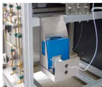
Acid pump for nitric acid
