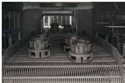
Mesh belt drive in a continuous furnace
